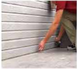
1. Draw a horizontal line on the wall. 安
