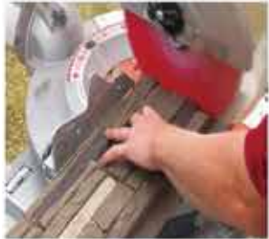
7. Cut the panel with a saw if necessary. 用手锯或电锯切割
