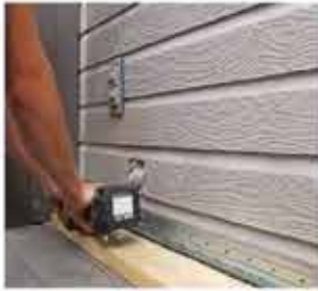
2. Put the starter strip on the bottom of the wall. 在墙底装水平条
