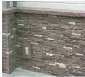
6. Keep on installing the panels, corners and top lines. 完成安装墙板、转 边
