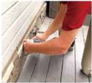
4. Lay the panels down to up, left to right, fix the panels with screws on the joints. 从左至右, 由下至上安装, 用螺丝固定
