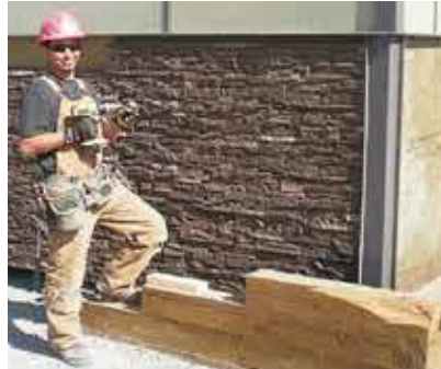
9. Upper panel interlocks with lower panel, screws are invisible 上板内扣下板, 安全牢固, 隐藏螺丝
