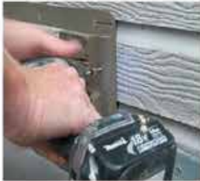
8. Drill the screw through the center of the joints to the wall 打螺丝的时候在舌边的中间打入
