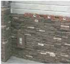
5. Check if the panels are horizontal with a level during installation. 安装过程中用水平尺测量是否平整
